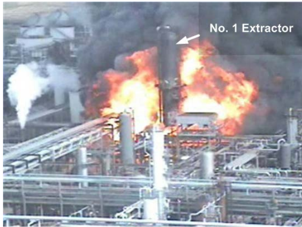
Figure 3 – Valero-McKee Refinery – 90 Seconds After Ignition.
