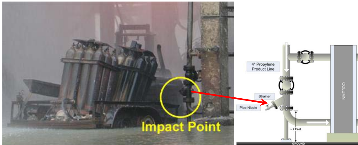
Figure 7 – Impact Point Showing Damaged Y-Strainer
